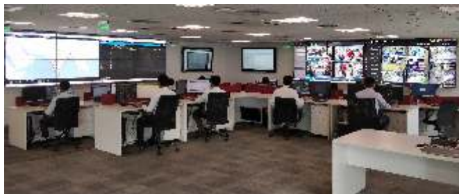
A view of the Bank's Command centre in Airoli, Navi Mumbai
